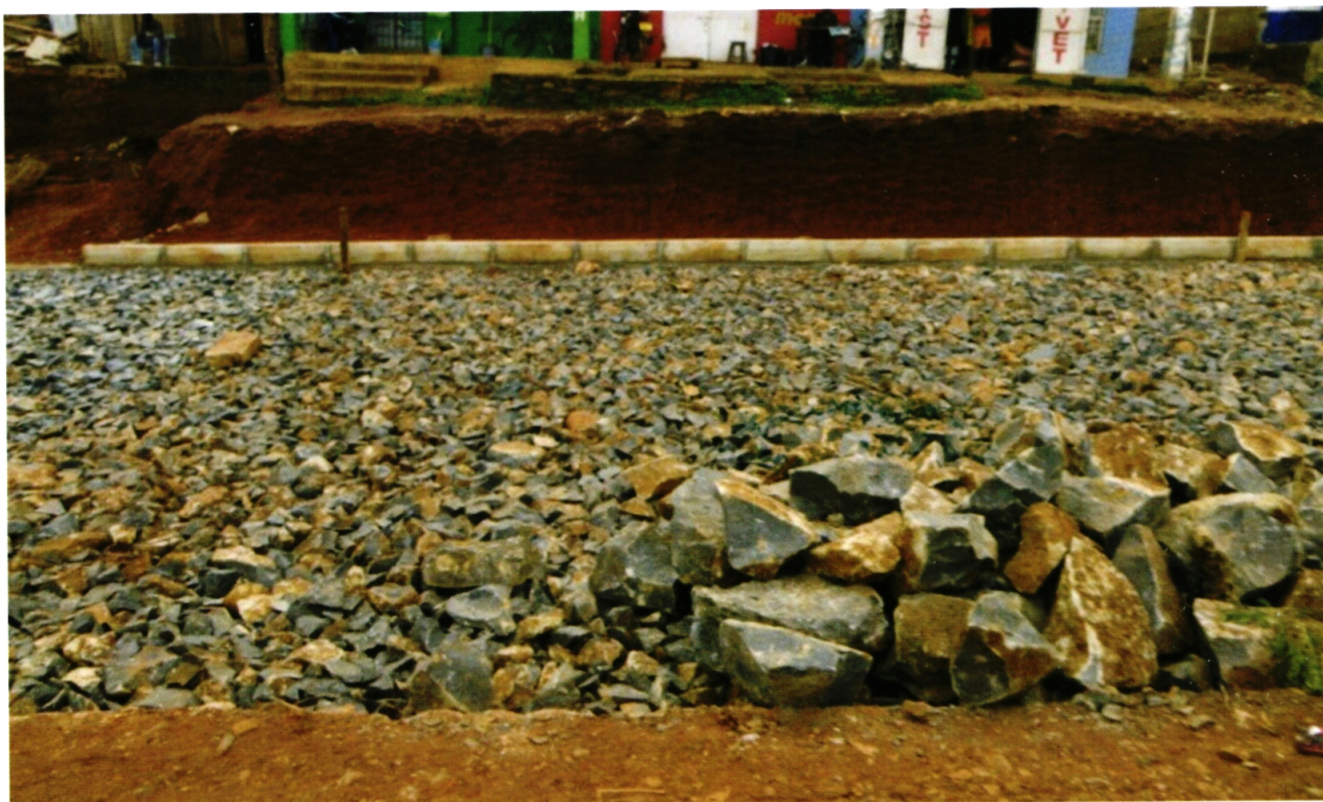
On-going road construction in West Pokot County.
