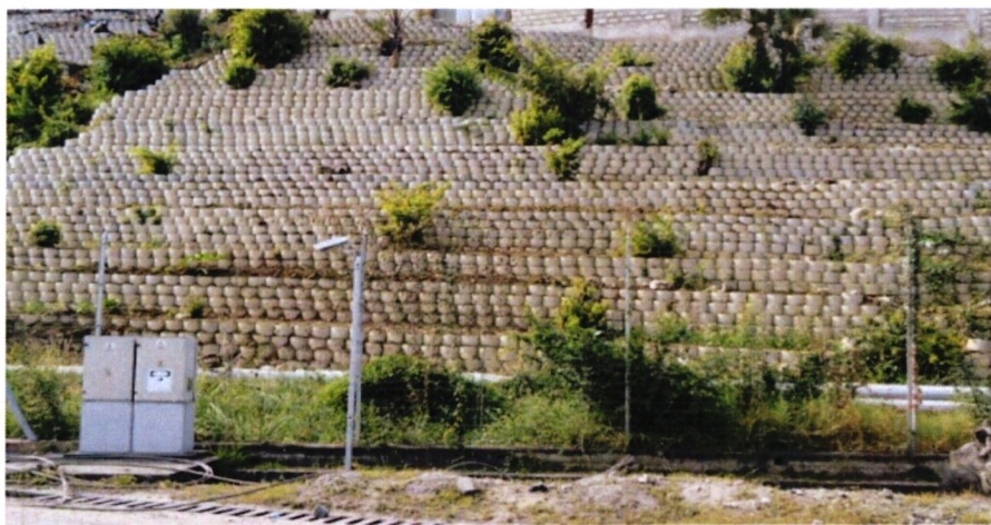
Site progress Photos
