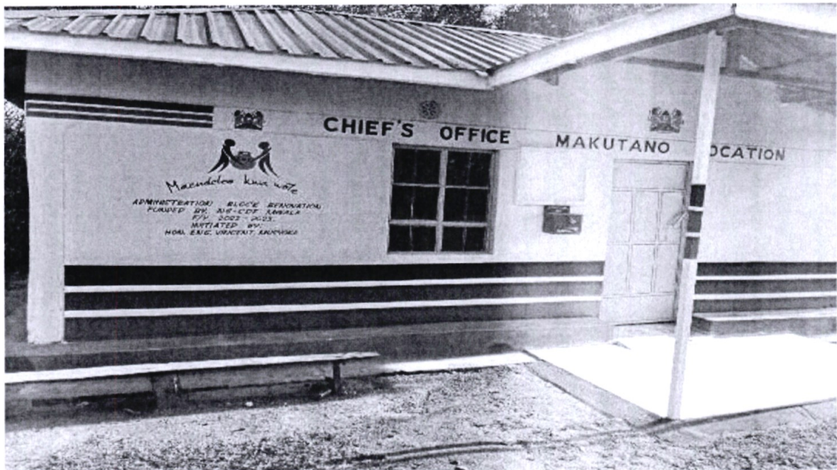
Makutano chiefs' office; Administration block renovation
