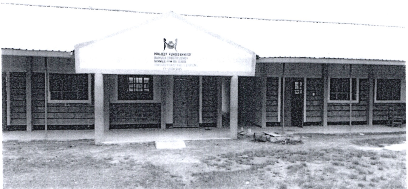
Figure 1: Construction of 4 No. Classrooms at Namanje FYM Primary School
