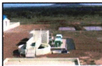
Aerial view of the ETP
