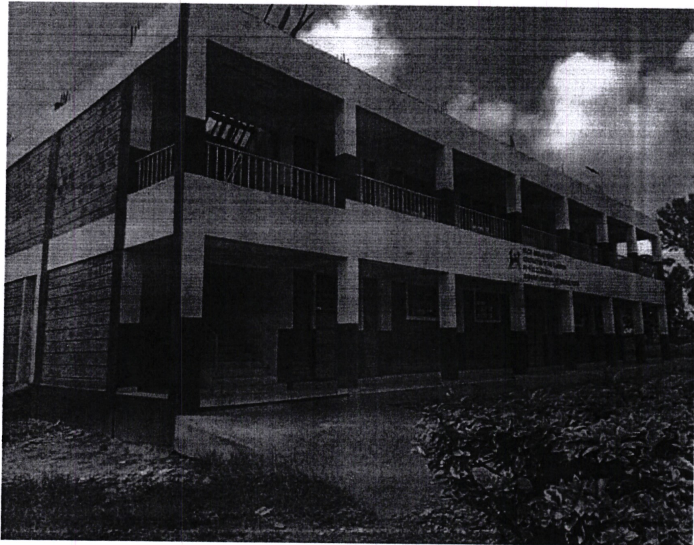
FIG 4: CONSTRUCTION OF FOUR NUMBER CLASSROOMS AT OURLADY OF FATIMA SECONDARY SCHOOL
