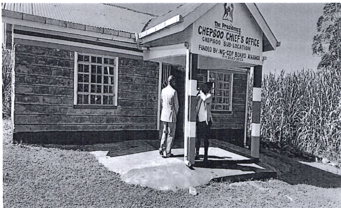
Chepsoo Chiefs office – Construction of chief's office
