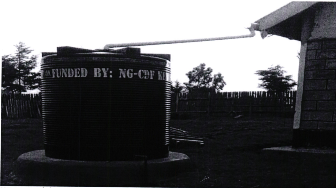
Water tank installed at Chebirei secondary school
