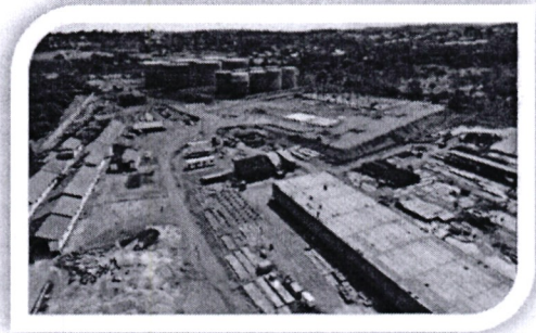
Aerial view of Mahathi Infra Jetty Facility in Bugiri-Bukasa, Entebbe – a complementary receipt jetty to KPC's KOJ.
