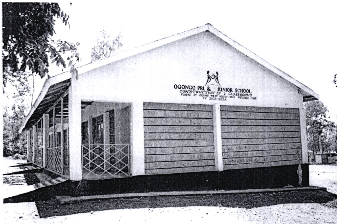
Fig 1.1 Construction to completion of 3 classrooms at Ogongo Primary and Junior School
