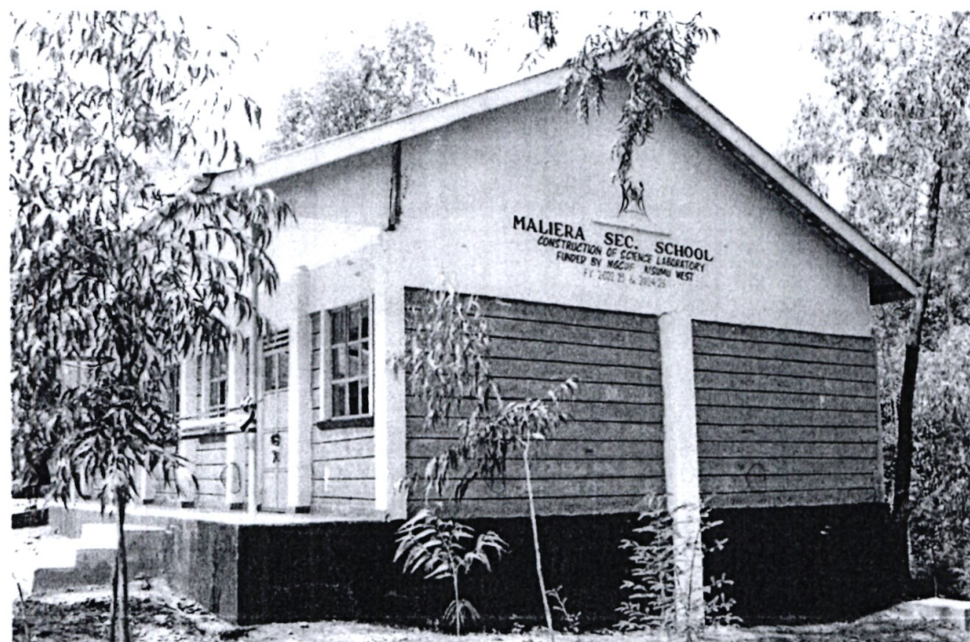
Fig 1.4 Photo of completed Science Laboratory at Maliera Secondary School
