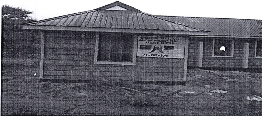
FIG 1.5 Enkaroni Primary School construction of a dormitory.
