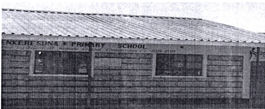
FIG 1.1 Enkeresuna Primary School construction of classroom.
