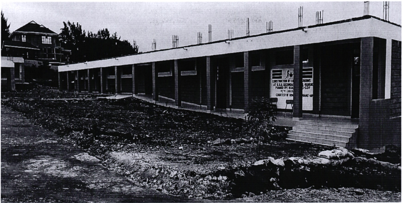
Construction of 4no. classrooms at GSU Secondary School.
