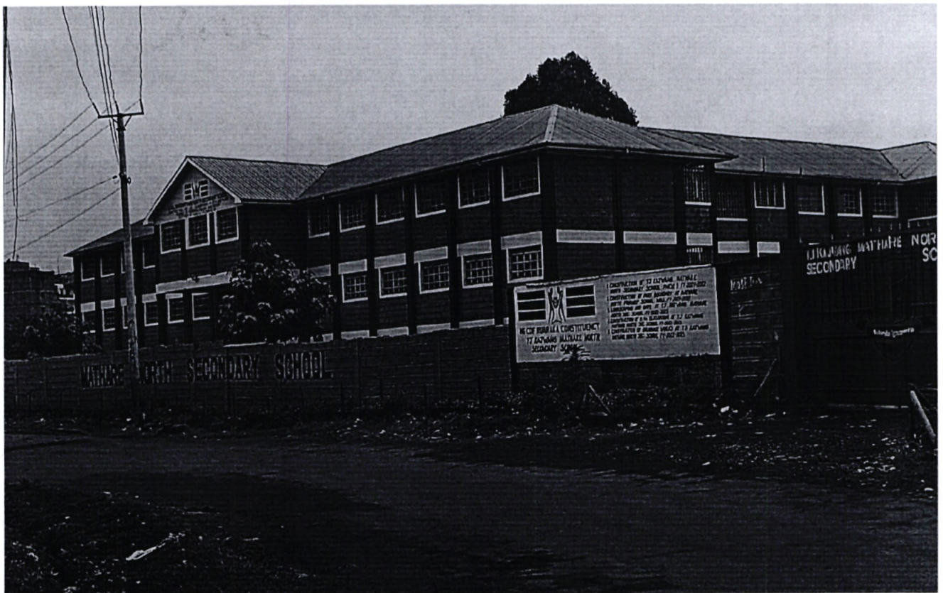
Construction of 24no. classrooms at TJ Kajwang Mathare North Secondary School.
