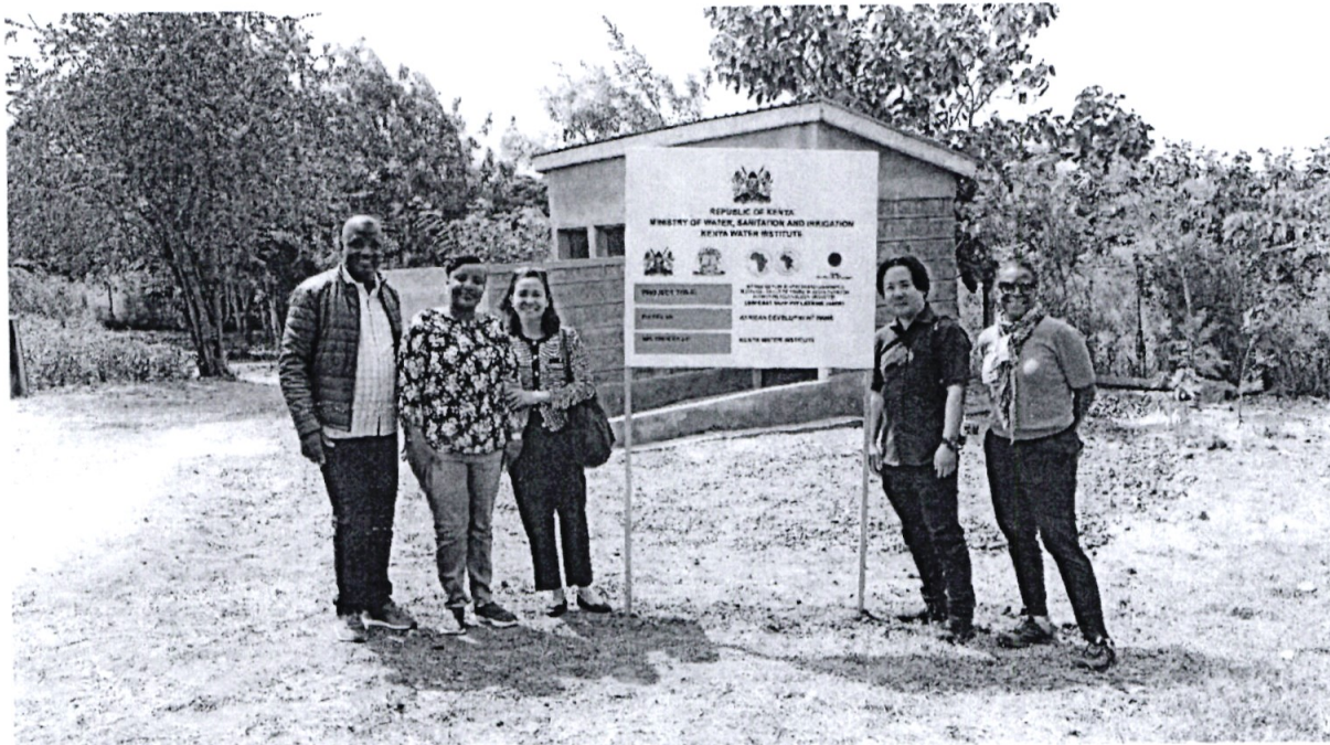
Mr. Nelson Kwamini, Deputy Director Research Consultancy and Technical Services leads an inspection committee of SATO toilets in Kitui County.
