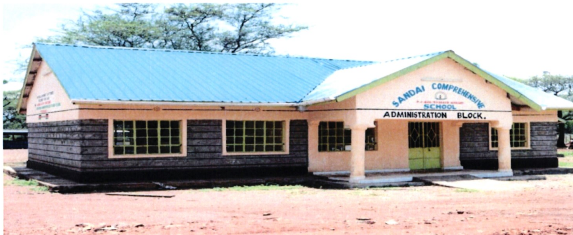
SANDAI COMPREHENSIVE SCHOOL: CONSTRUCTION OF ADMINISTRATION BLOCK
