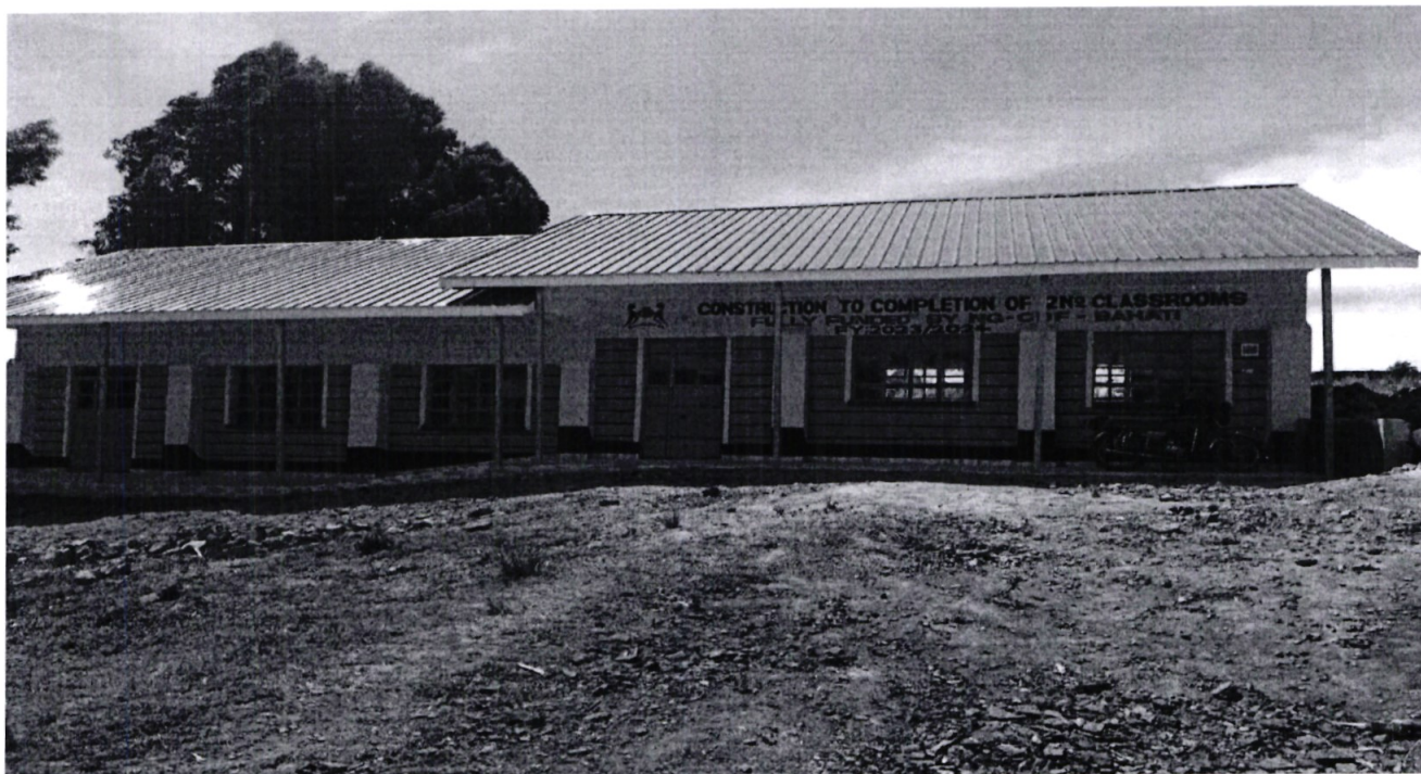
Construction of two classrooms at Kimani Ngunjiri Primary School
