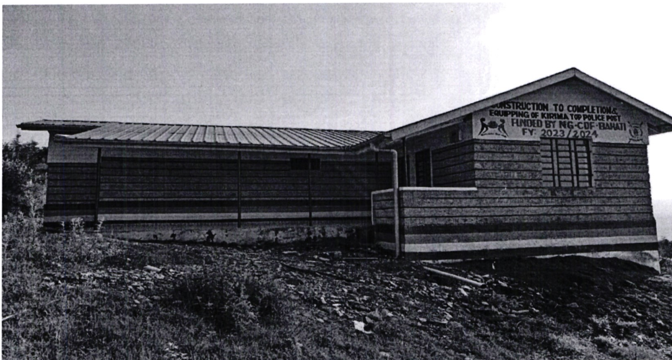
Construction and equipping of Kirima Top Police Post
