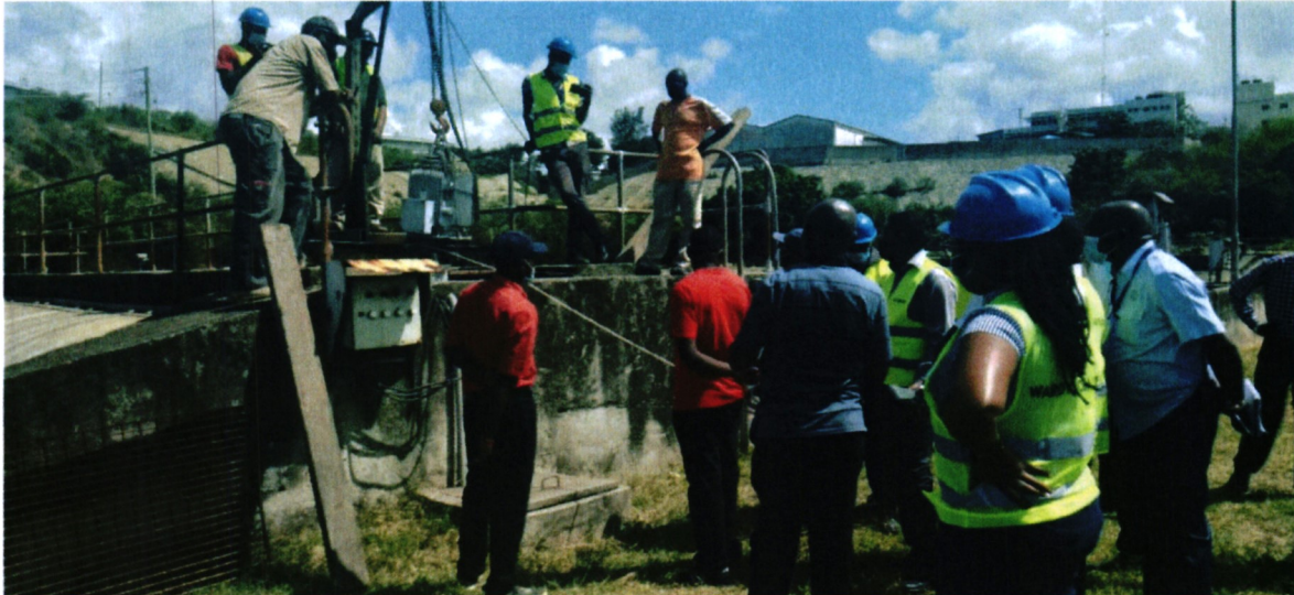
A multi-Agency joint inspection of the Kipevu sewage treatment plant on June 2nd 2021
