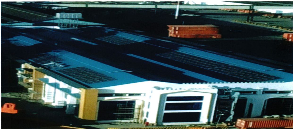
Roof top Solar panels at the Cruise ship terminal
