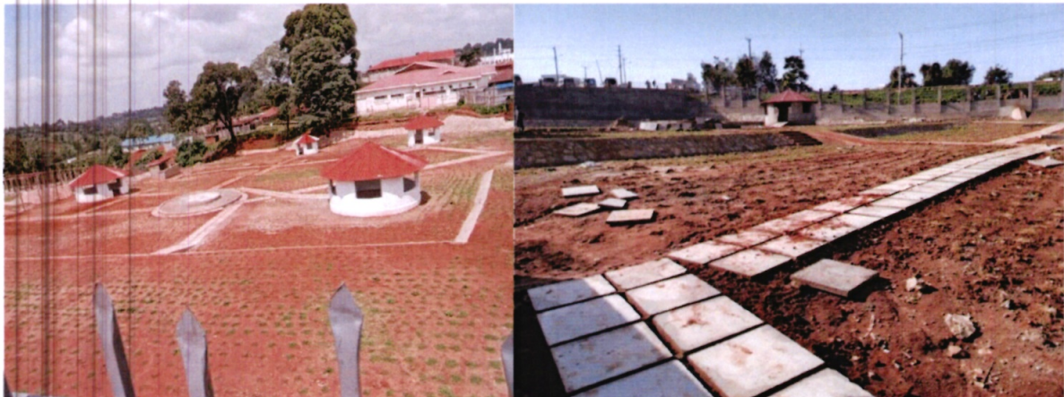
Figure 1: Ongoing construction of Makutano recreational park
