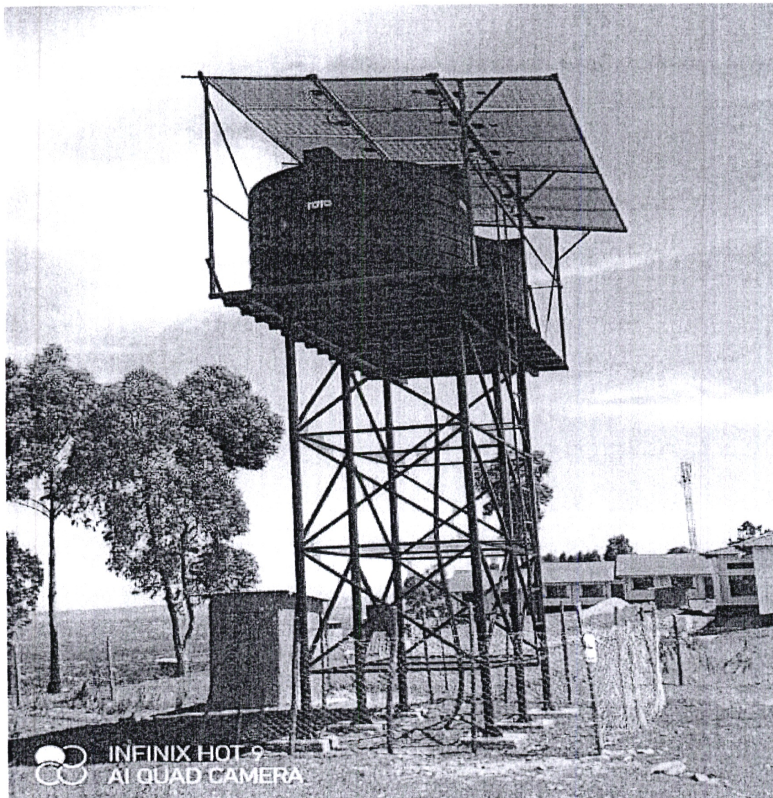
RAMBA PRIMARY SCHOOL WATER PROJECT AND RENOVATED CLASSROOMS,
