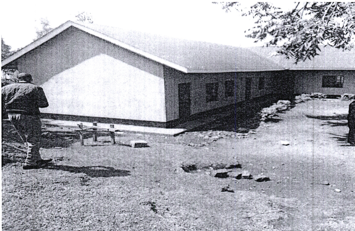
RENOVATED 4 CLASSROOMS AT KENYAMBI PRIMARY.
