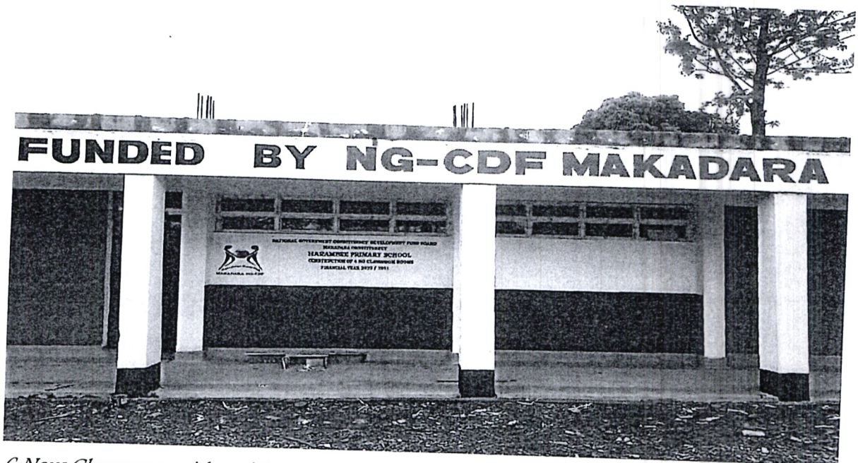
6 New Classroom with a slab at Harambee Primary School
