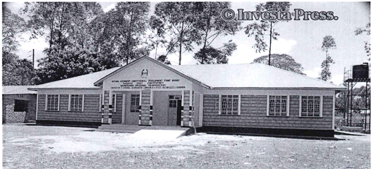
Fig 4: Completed Security Project at Namarambi Assistant County Commissioner's Office.
