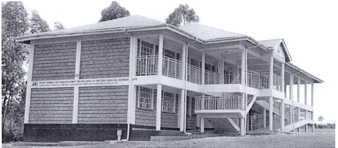
Fig 3: Completed Admin Block Cum Library at Bakisa Girls Secondary School.
