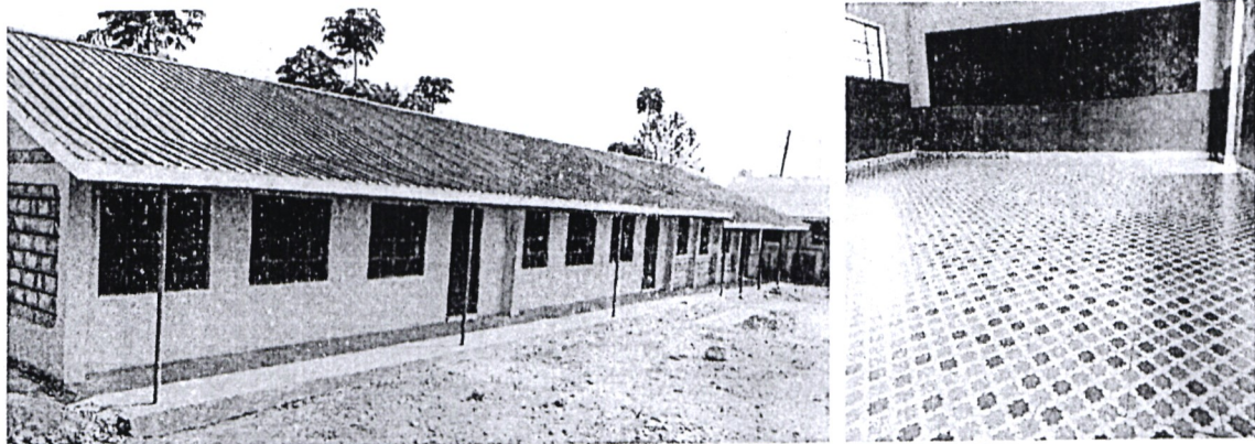
MUKURWE WA NYAGATHANGA SECONDARY SCHOOL NEW CLASSROOMS
