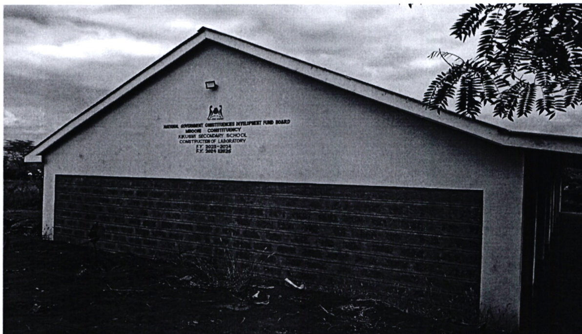
(Construction and equipping of Kikuswi Secondary School 50 students' capacity science laboratory)
