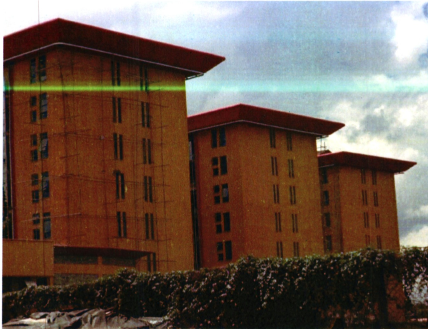
The New Mitihani House (Ongoing Project)
