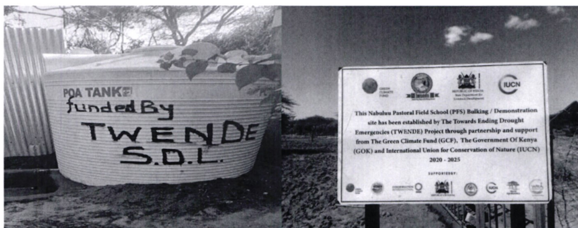
i. Wamba Disabled Group tank
