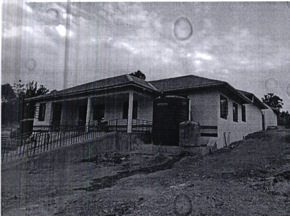
Pic. 5: Gambogi modern Police Station newly constructed fully funded by Hamisi NG-CDF
