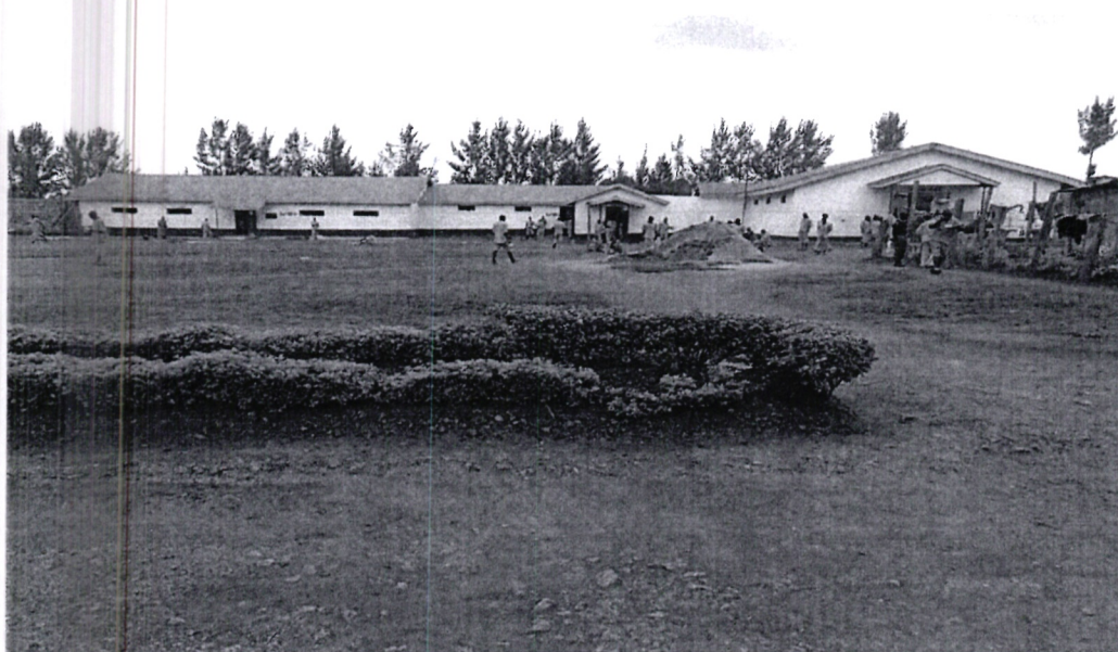
Ngeria prison: Completed Mixed block
