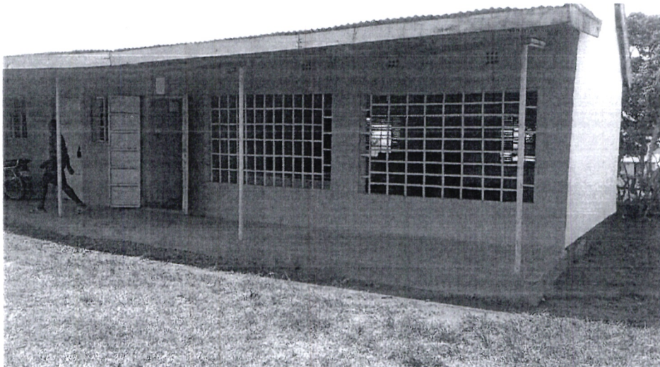
Shikusa Borstal Institution: Completed Welding Workshop
