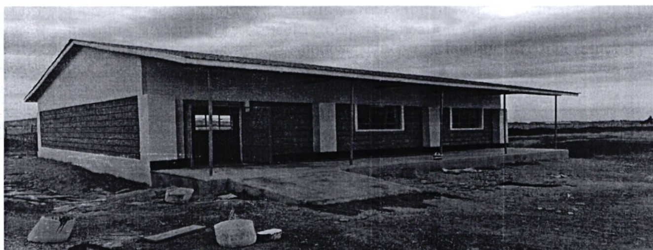
FIG 2: MALILI TOWNSHIP PRIMARY SCHOOL
