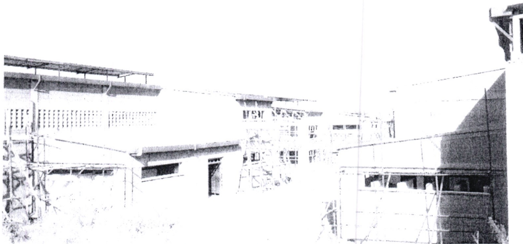
Front view of 4 small warehouses at 85% complete
