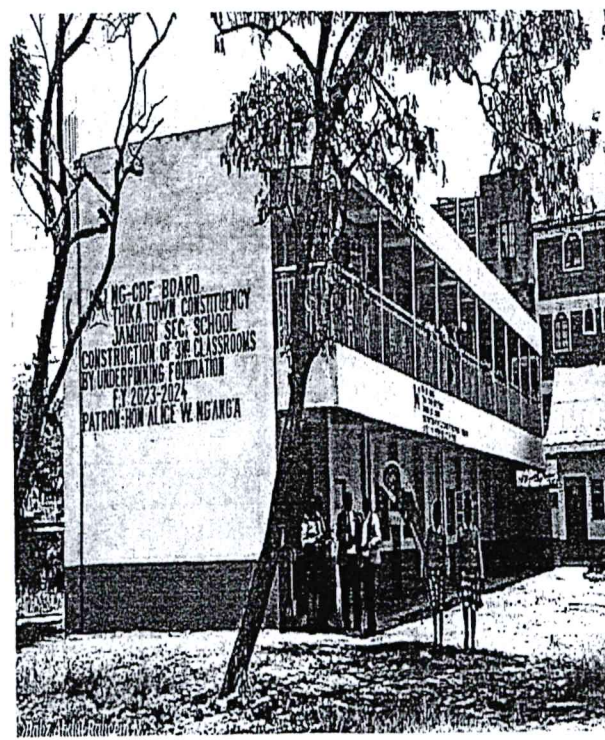
3no. classrooms at Jamhuri Secondary School through underpinning foundation (complete)
