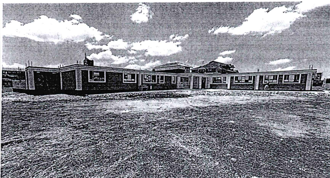
Ngoing'wa Police Station Phase 1 complete, phase 2 ongoing
