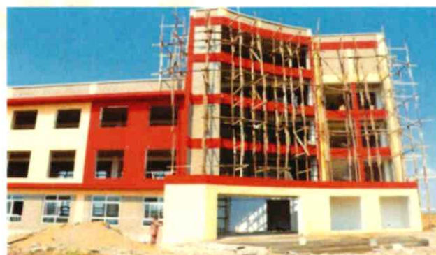
The One-Stop Shop/Administration Building under construction
