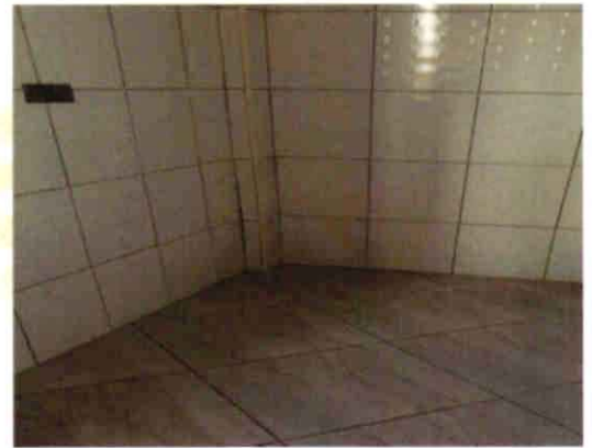
Ongoing tiling of internal common areas
