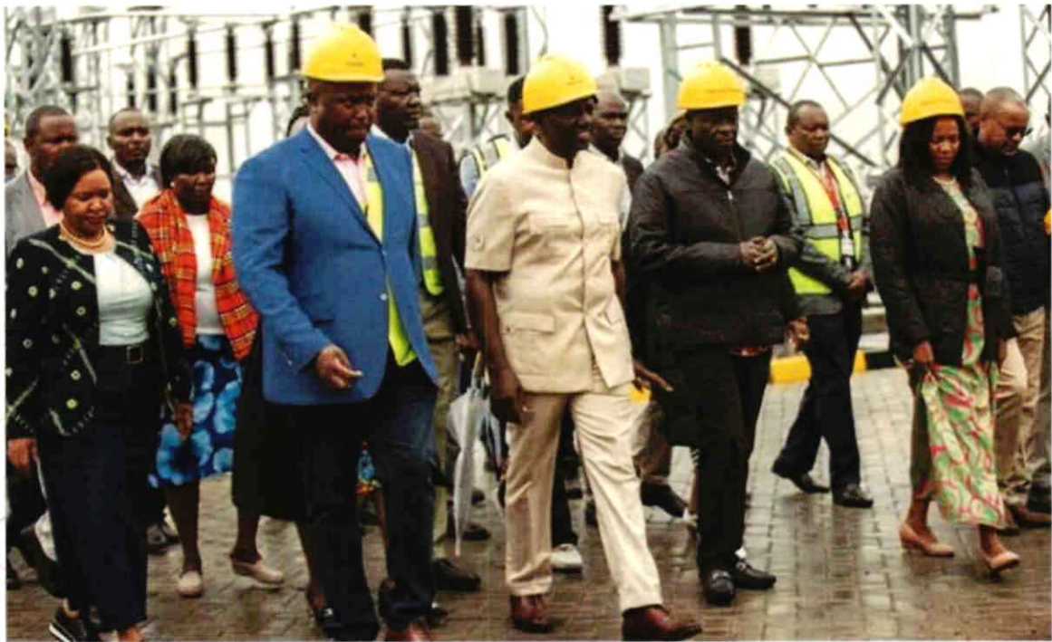
H.E. The President Dr. William Ruto inspecting the power sub-station at the Naivasha SEZ
