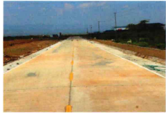
Completed and marked road section of the Access Road 2 leading to Jumbo AAA SEZ Ltd
