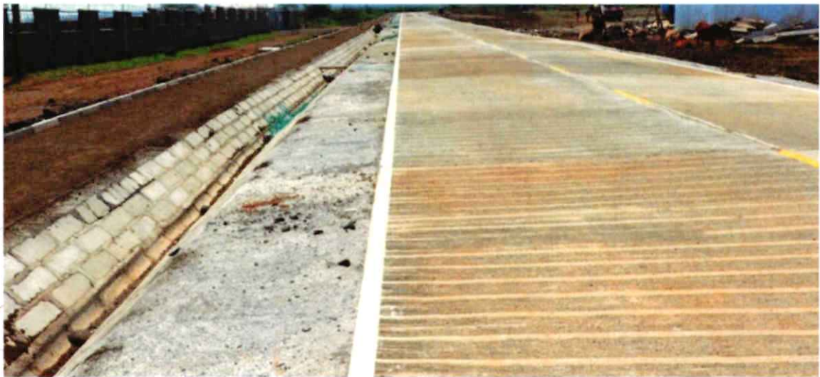
Completed Pedestrian footpath, side drain, shoulder and Concrete pavement
