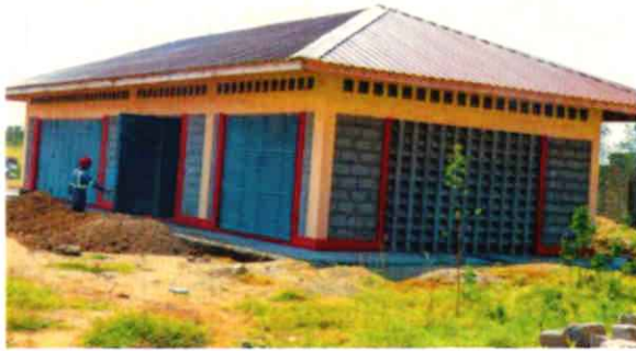
The Generator/Power house under construction
