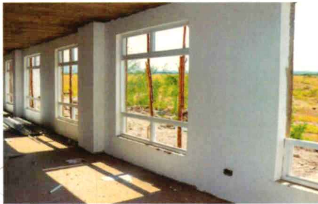
Ongoing fitting of windows
