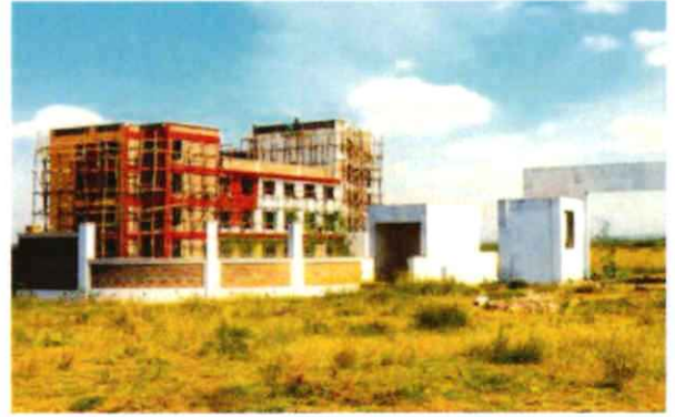
The gate under construction
