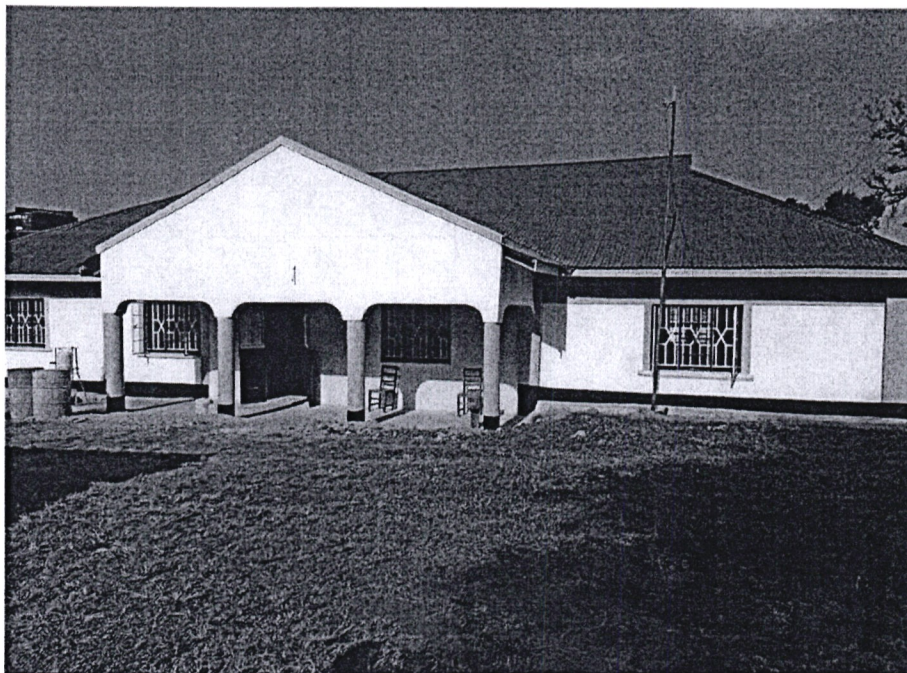
3. CONSTRUCTION OF DEO'S OFFICE F/Y 2019/2020
