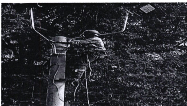
Installation of high mast street lights
