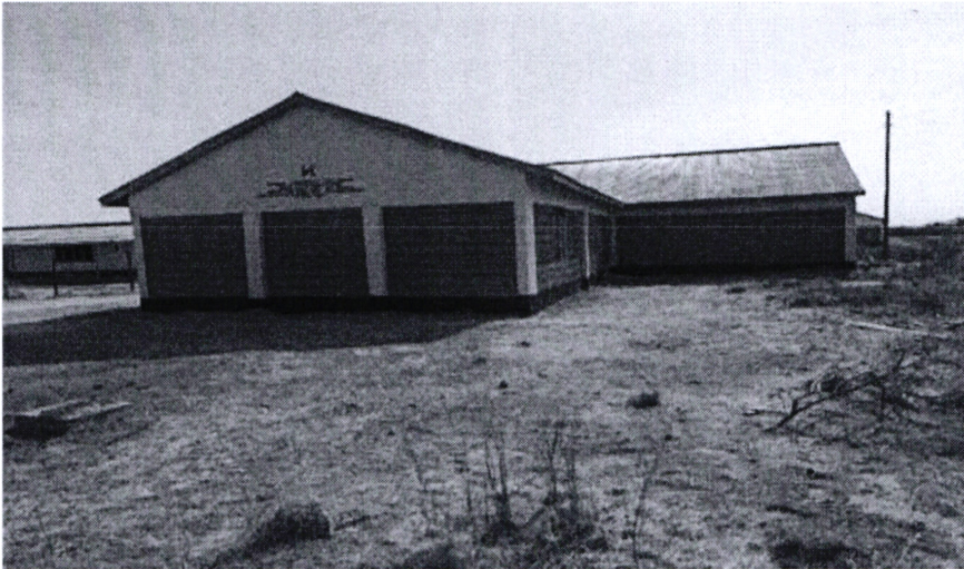
Senior Chief Ogle Girls Secondary School: Construction to Completion of Dining Hall and Kitchen.
