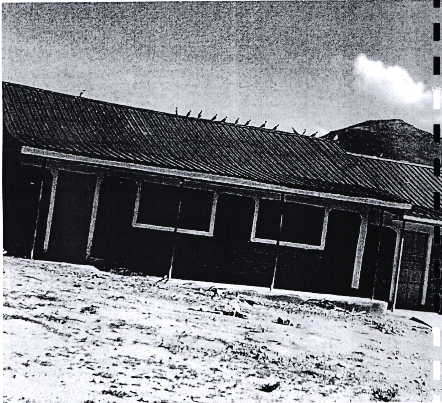
2classrom construction at morijo mix sec school
