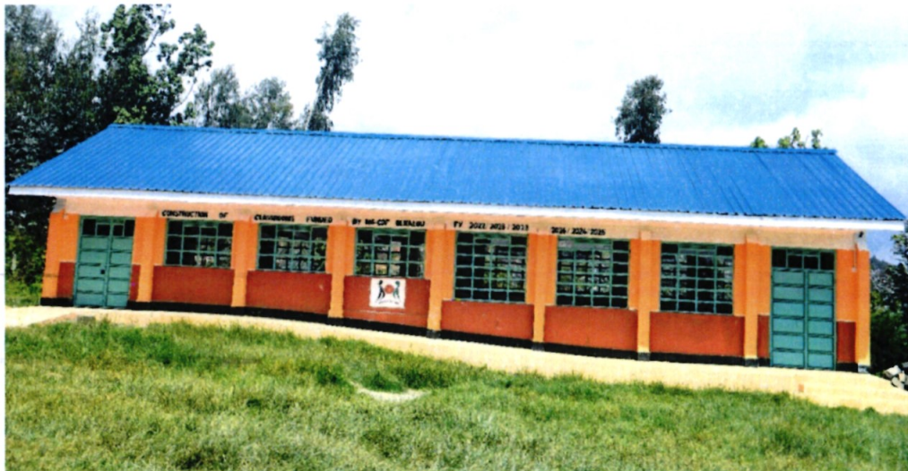
Construction of 2 classrooms at Kahonge primary school
