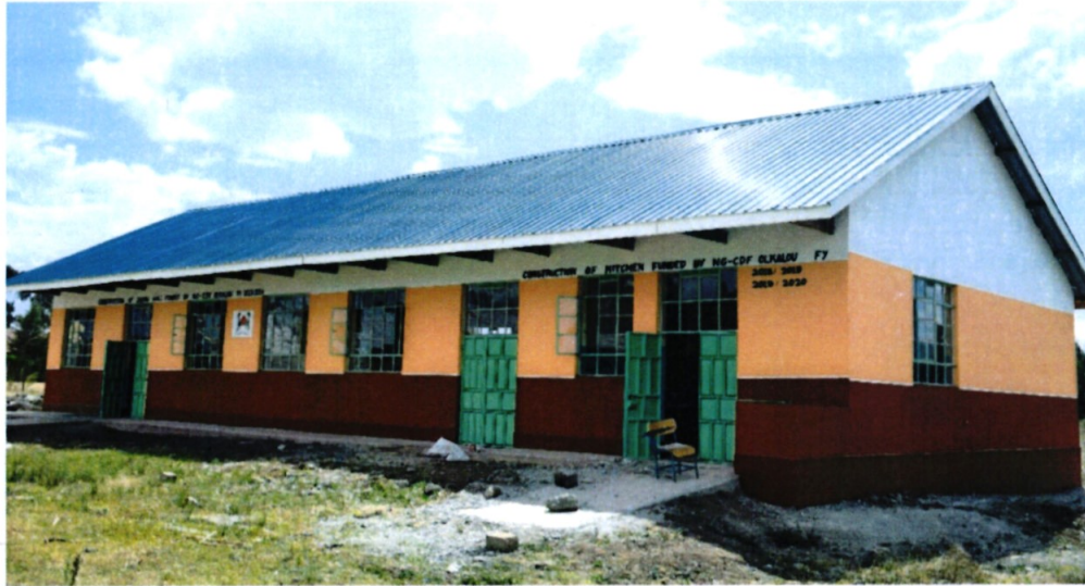
Construction of a multipurpose hall and kitchen at Mukindu secondary school
