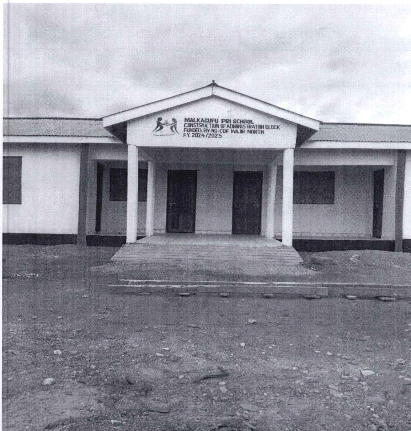
Malkagufu Primary School: Construction to completion of one block of 4 staff rooms
