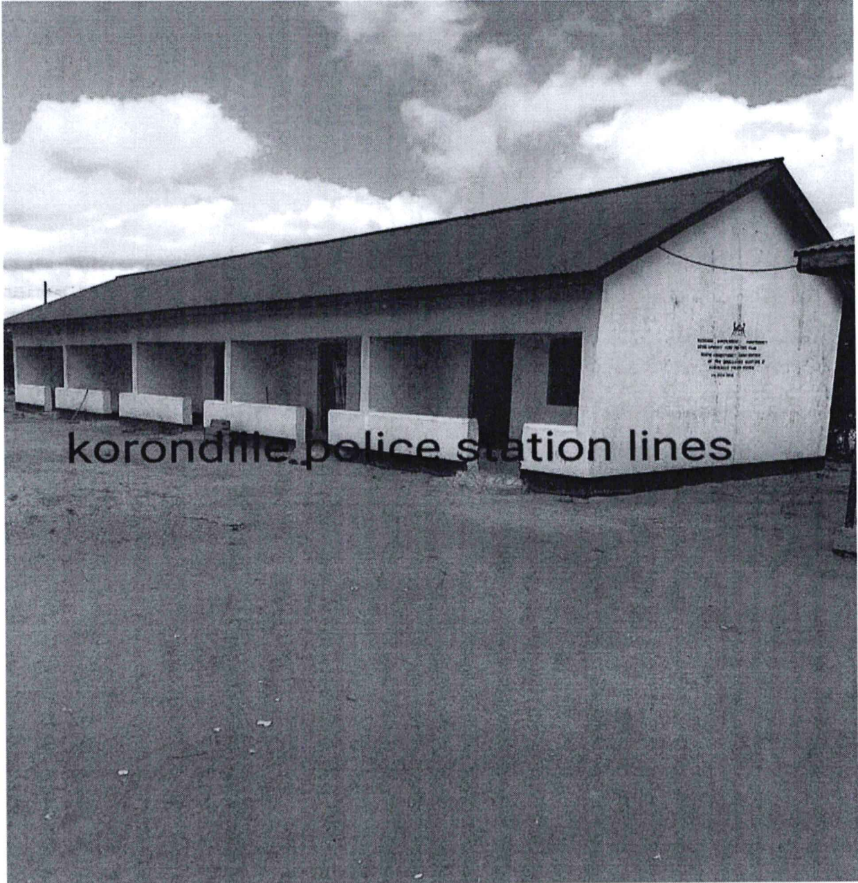
Construction to completion of a block containing five single-room units
