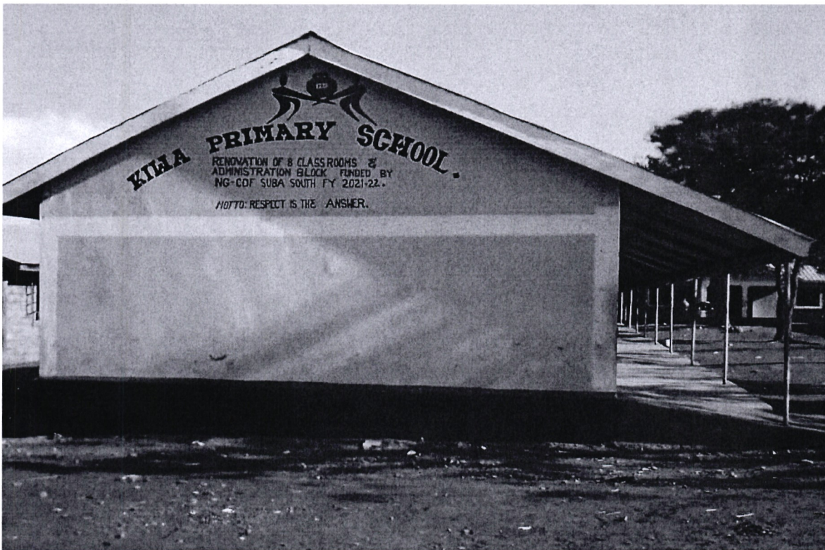
Kiwa Primary School: Renovation of 8 classrooms and administration block Funded: FY 2021-2022: Allocation Ksh 1,200,000 FY 2021/2022
