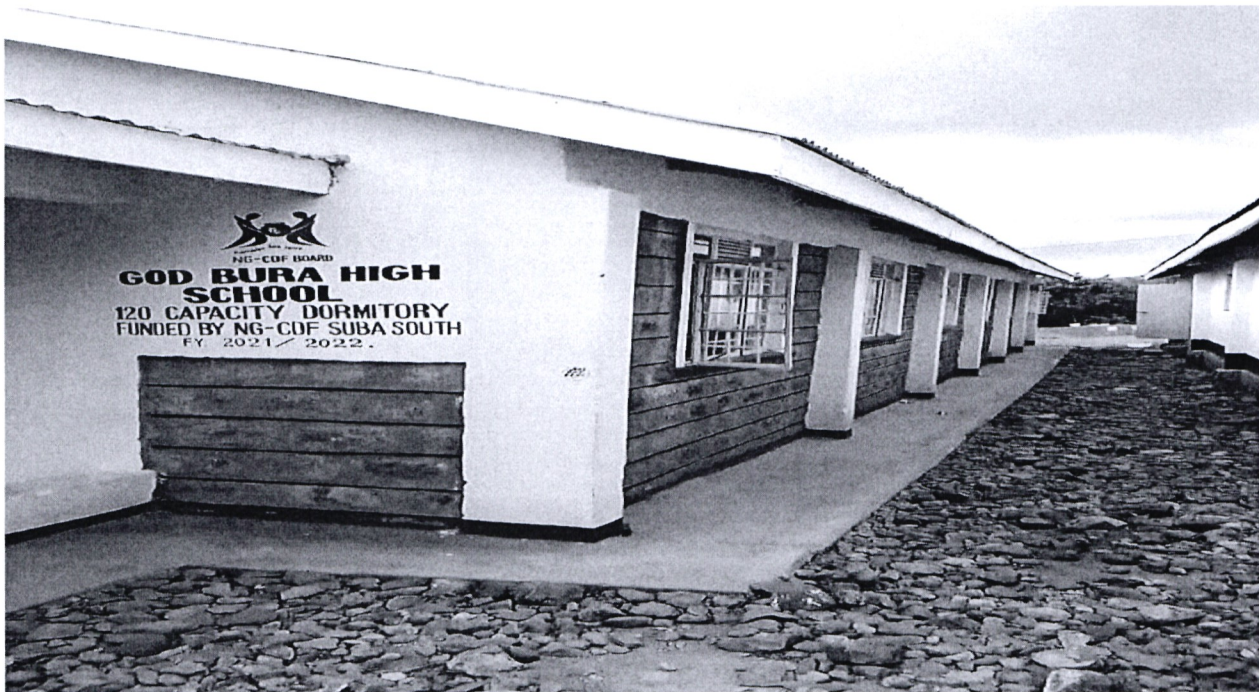
God Bura Secondary School: Construction of 120 capacity dormitory: Allocation Kshs 4,000,000 FY 2021-2022
