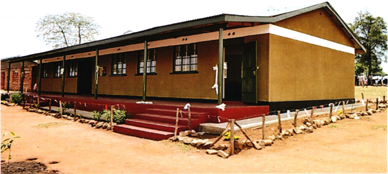
Administration Block constructed at Ndururumo Secondary School- Laikipia County
