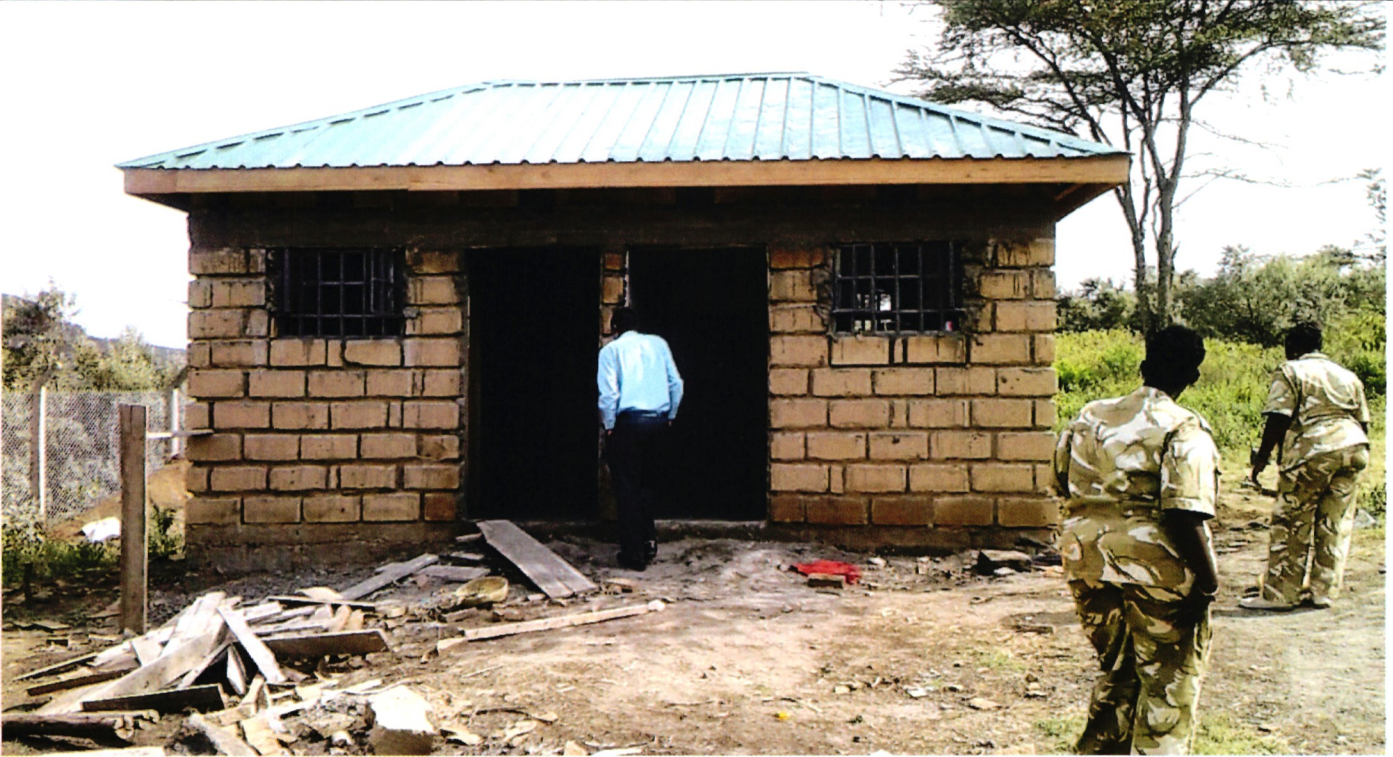
The Narasha community ablution block in progress.
