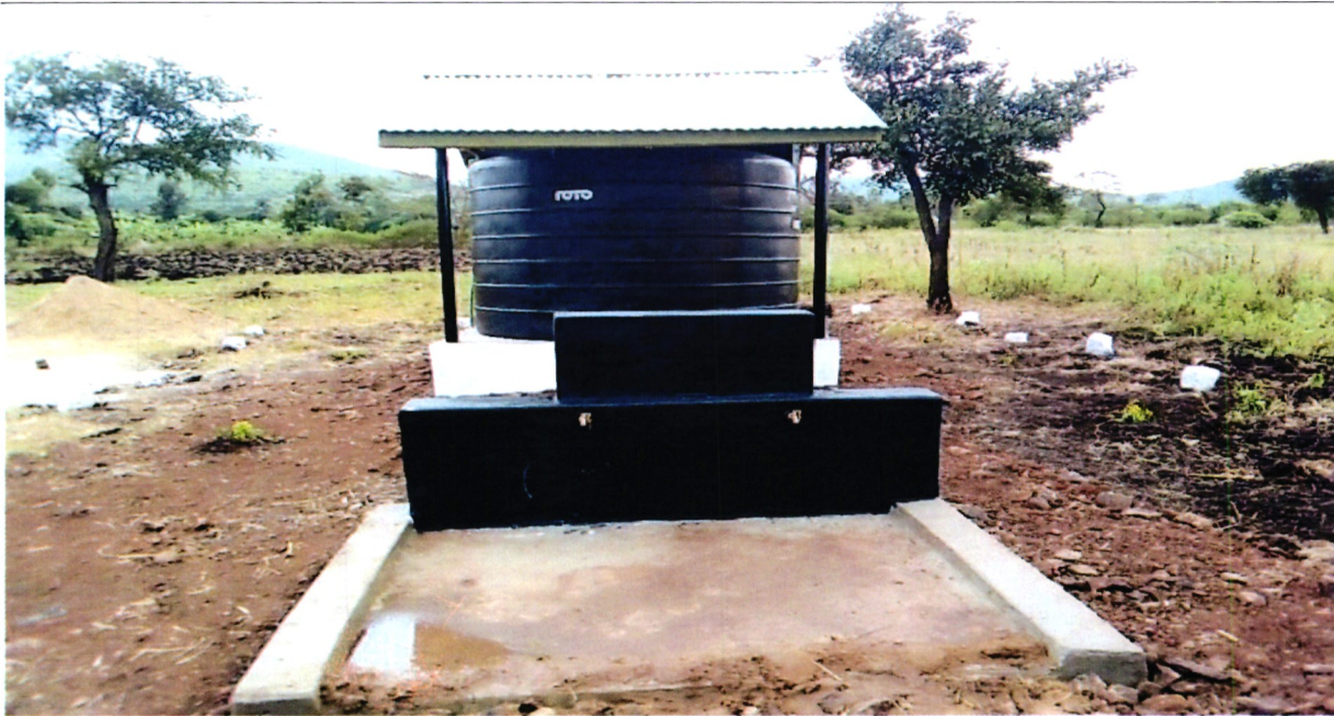
A 10,000 litre water tank installed for Nyadenda community
