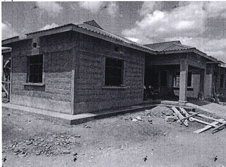
g) On-going Construction of Administration Block at Fayya Girls secondary school.
