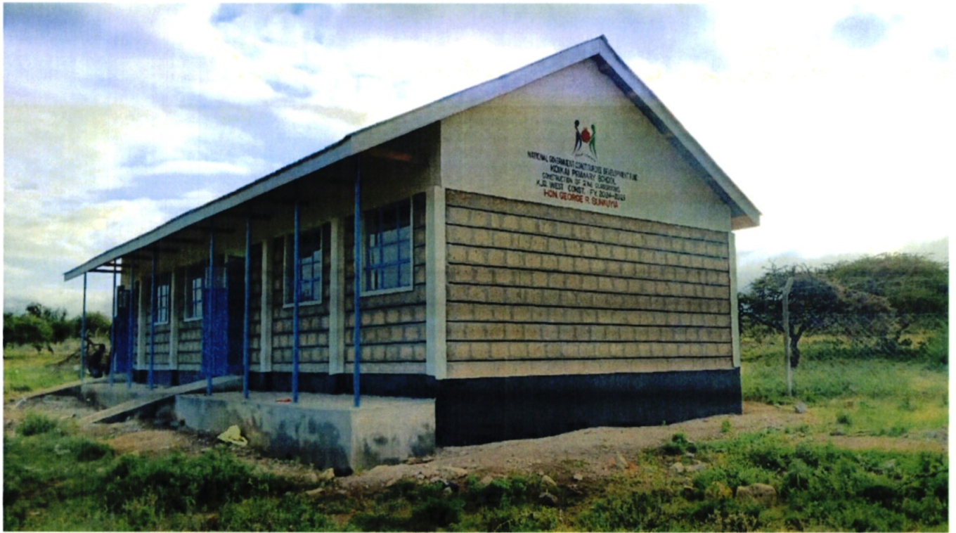
OLCHORO ONYORI DAY SECONDARY SCHOOL CLASSROOM CONSTRUCTION
