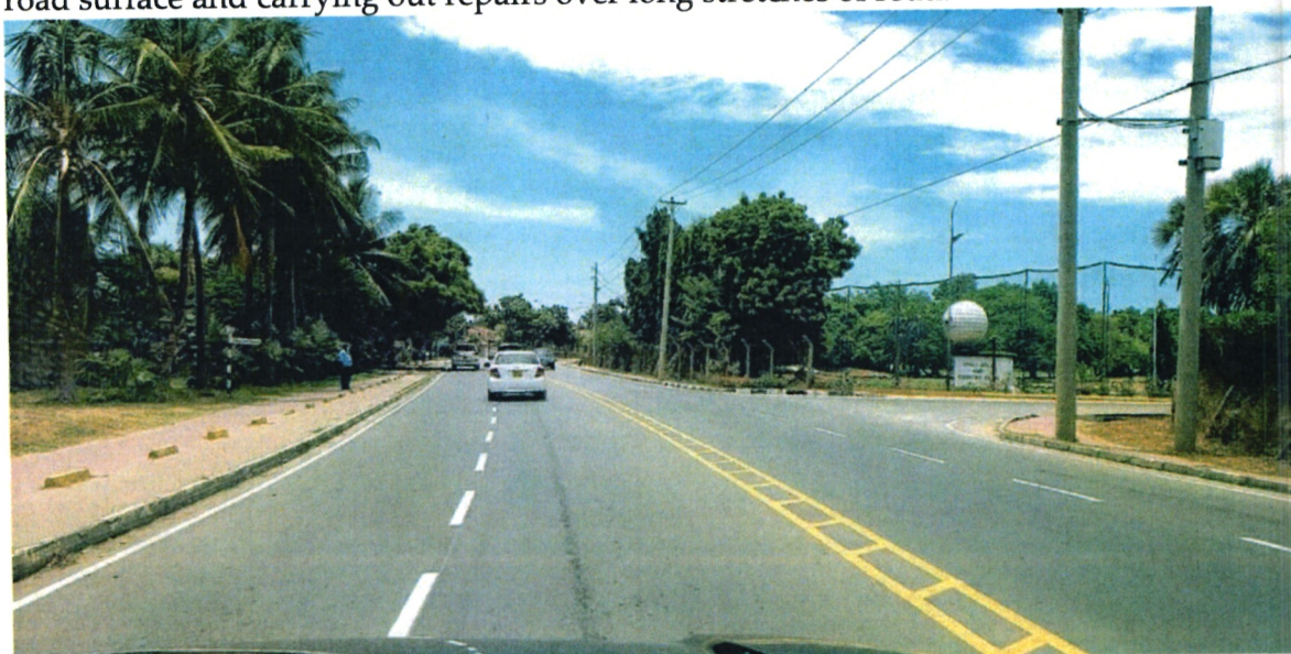
Figure 8: Rehabilitation of Links Road Nyali , Mombasa County
