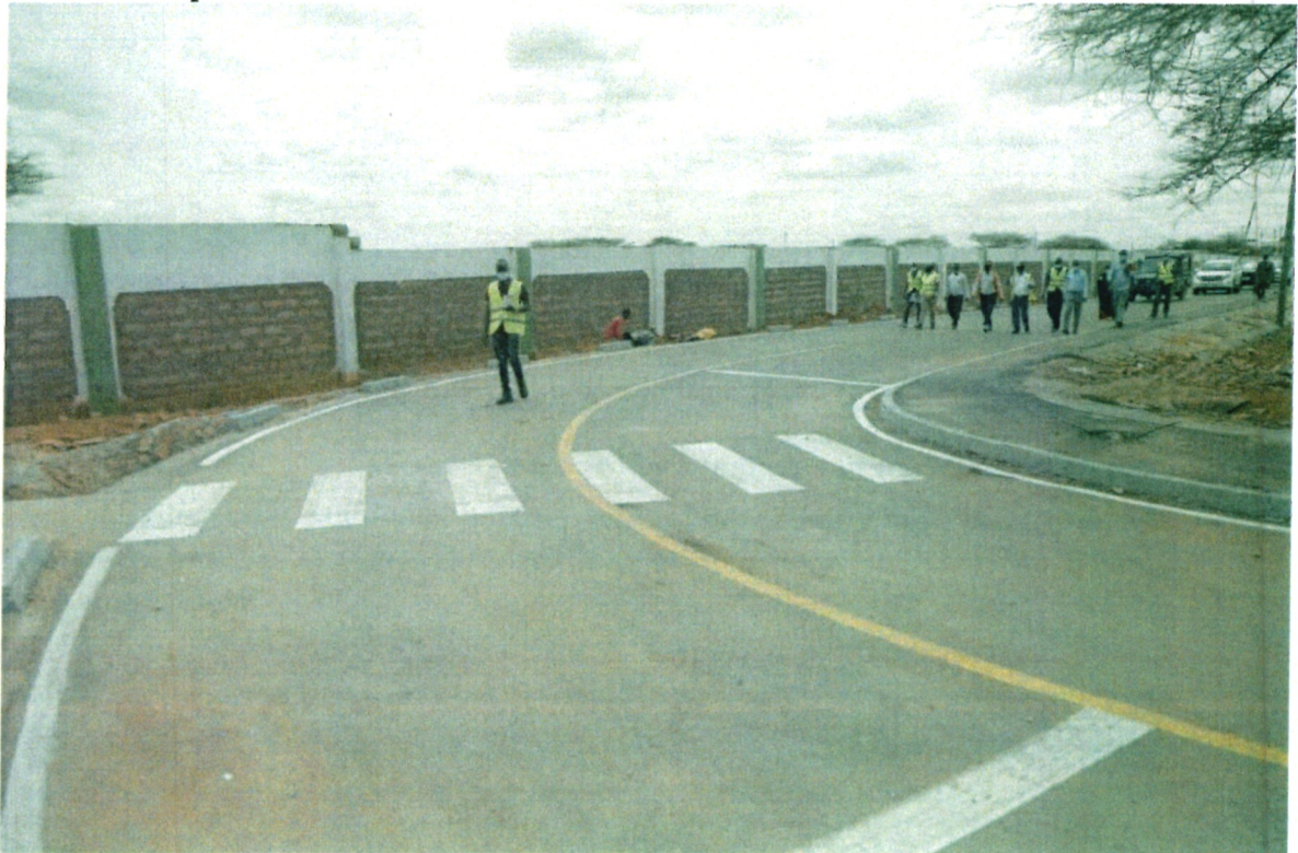
Figure 10: Quality Control - Inspection of works during substantial inspection of Mandera Town Roads
