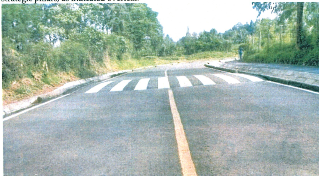
Figure 2: Completed section of Kericho Bypass
