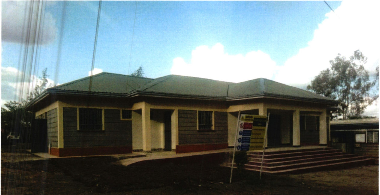
Newly constructed Samburu Office
