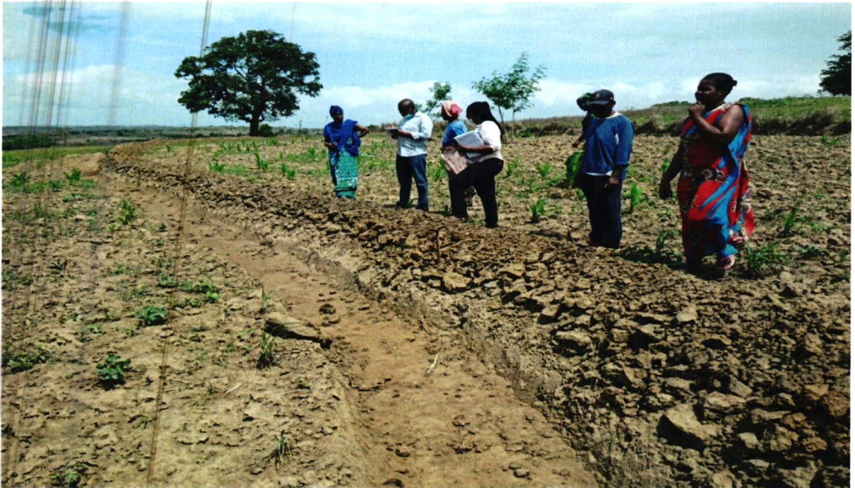
Ongoing terracing work at Mwache
