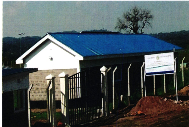
Chain-link fencing and farm house construction at Lichota Integrated Technology Transfer Centre
