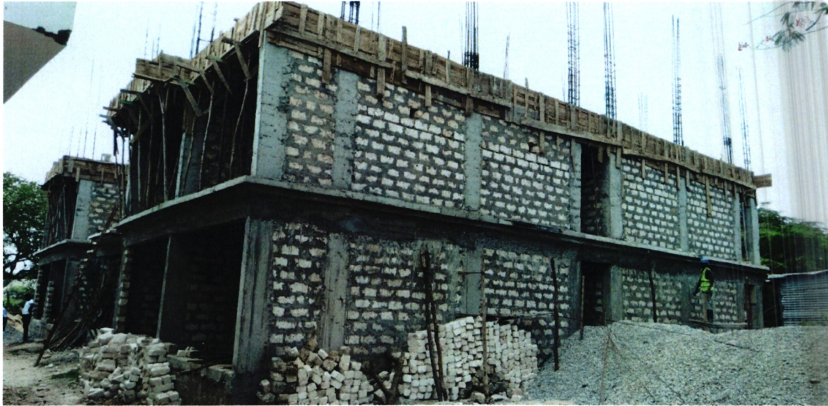
Construction of accommodation room in progress
