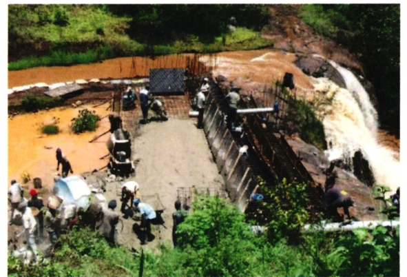
Gaitega Gaturi project-River diversion works during intake structure construction
