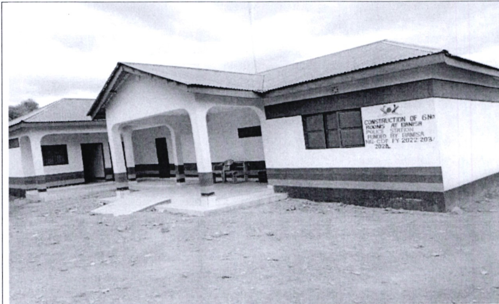
Banisa Police Administration Office newly built and in use. This has enhanced service delivery.
