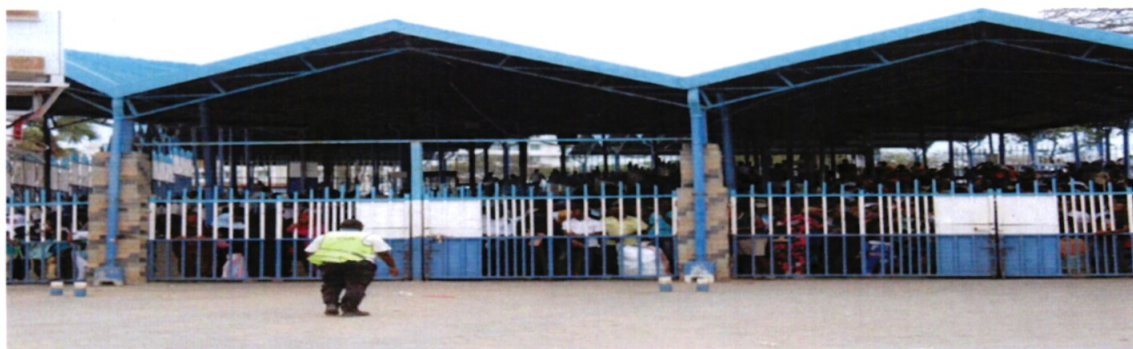
Likoni Ferry passengers holding area.
