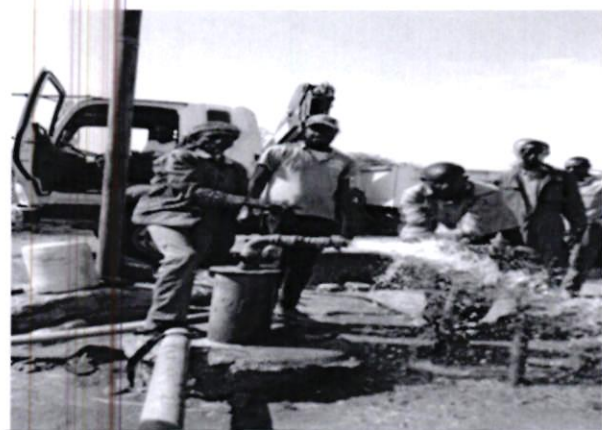
Borehole Drilled in Belgesh
