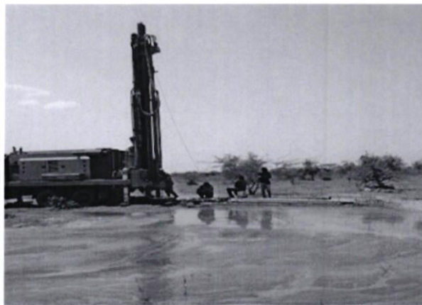
Drilled Borehole in Cherab Ward
