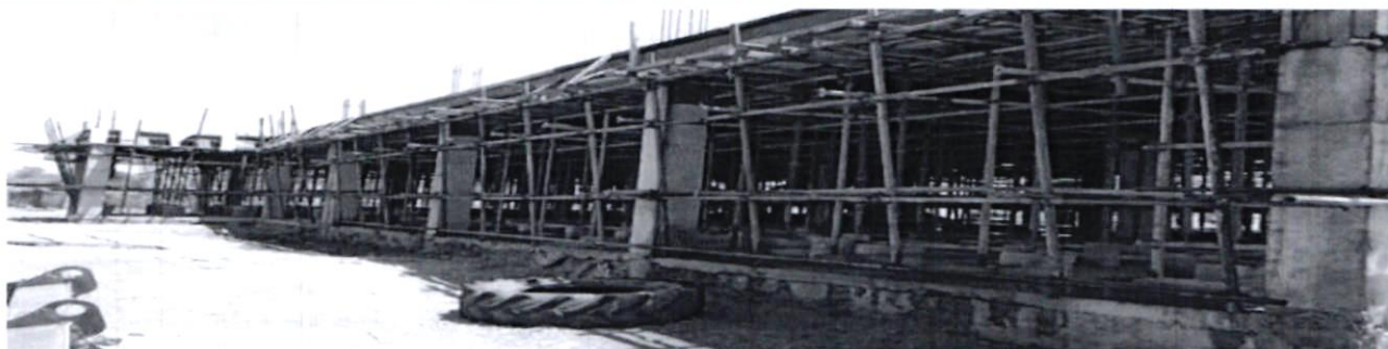
Isiolo County Modern Market under Construction
