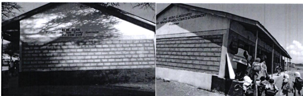
ECDE Classrooms in Merti Sub County
