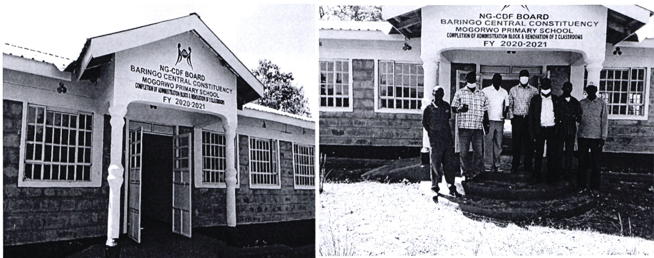
Mogorwo Primary School – Construction And Completion Of 1 Administration Block
