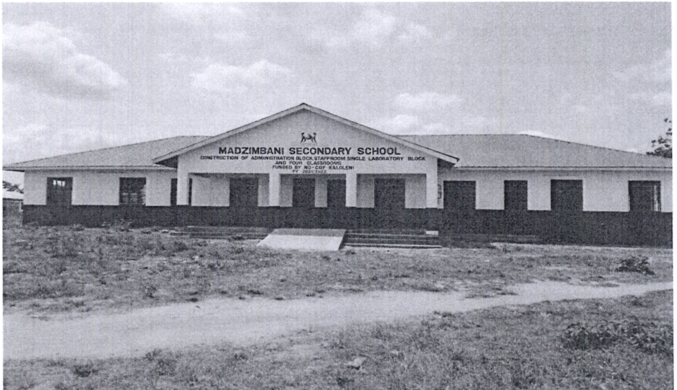
Madzimbani Secondary School: Construction to completion of an Administration block and 4 no classroom and 80 students capacity Laboratory.
