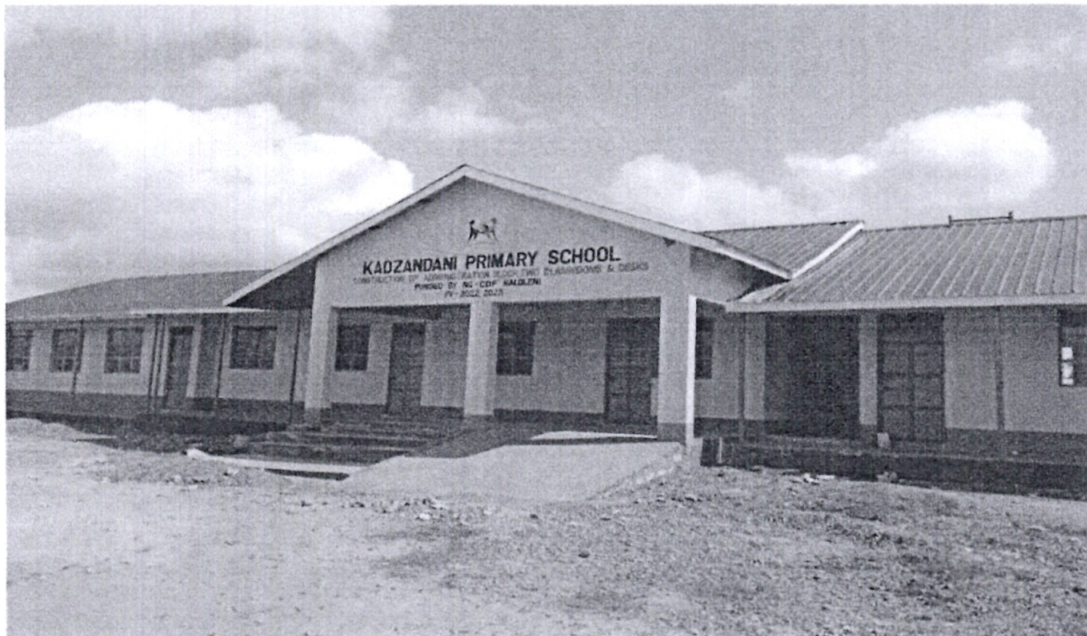
Constructed Administration block and 2No. Classrooms at Kadzandani Primary School
