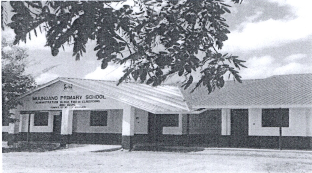
Constructed Administration block and 2No. Classrooms at Muungano Primary School
