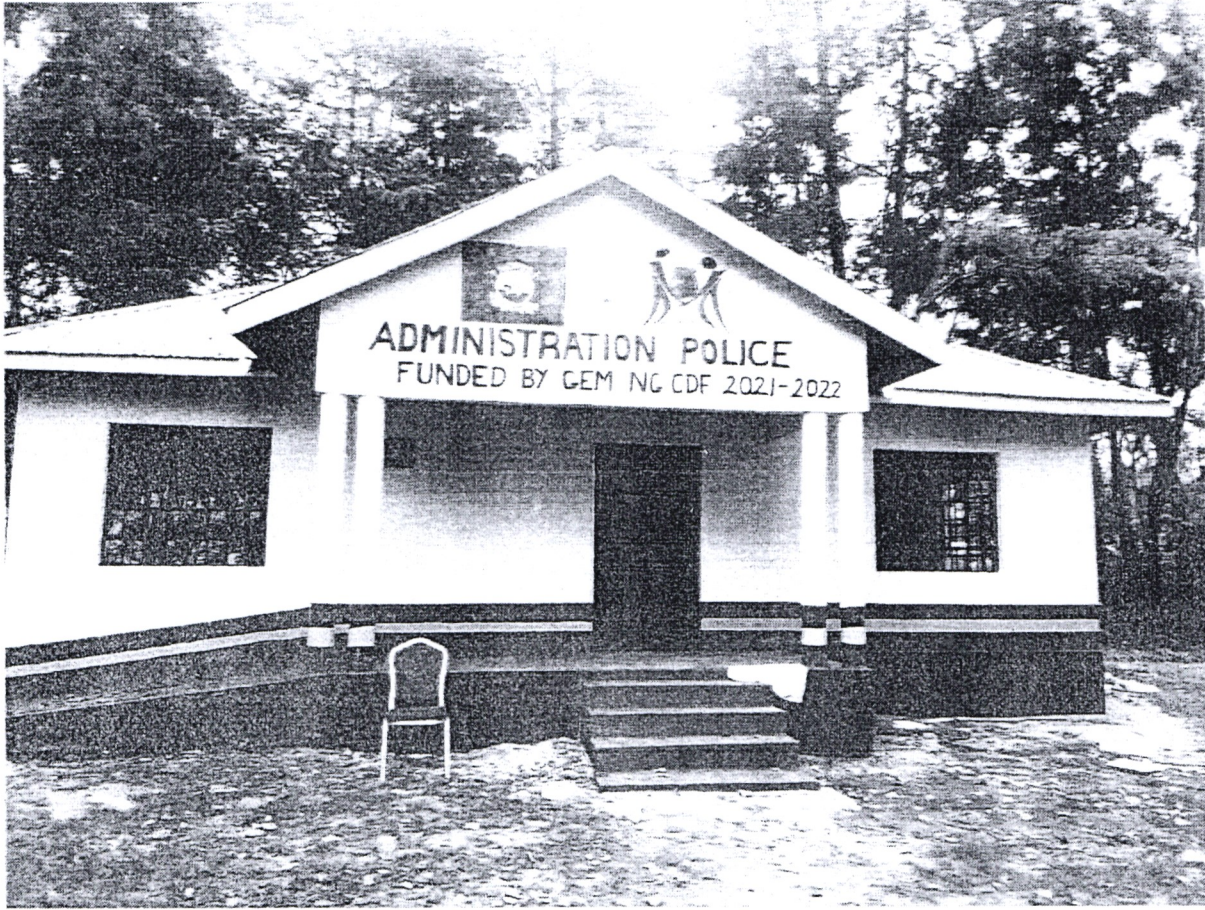
Gem Yala Sub-county AP Commandant's office constructed at a cost of Kshs. 1,000,000.00
