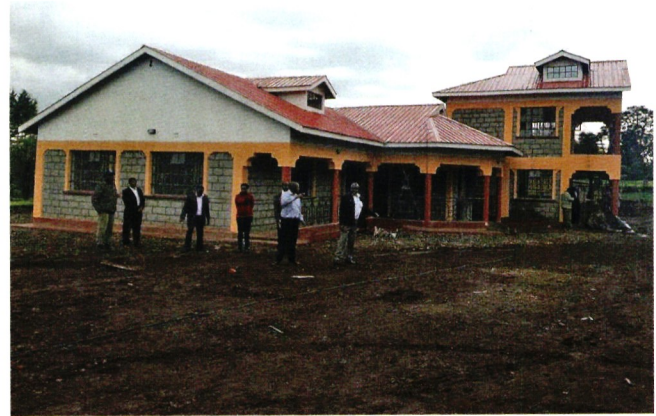
Kaminjeiwet Resource Centre in Kericho County that has been constructed by KPC Foundation.
