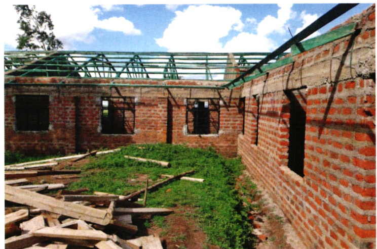
Ongoing construction of administration block and classes at Masangora Girls Secondary School.
