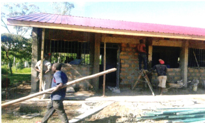
Ongoing construction works at Simbi Secondary School.
