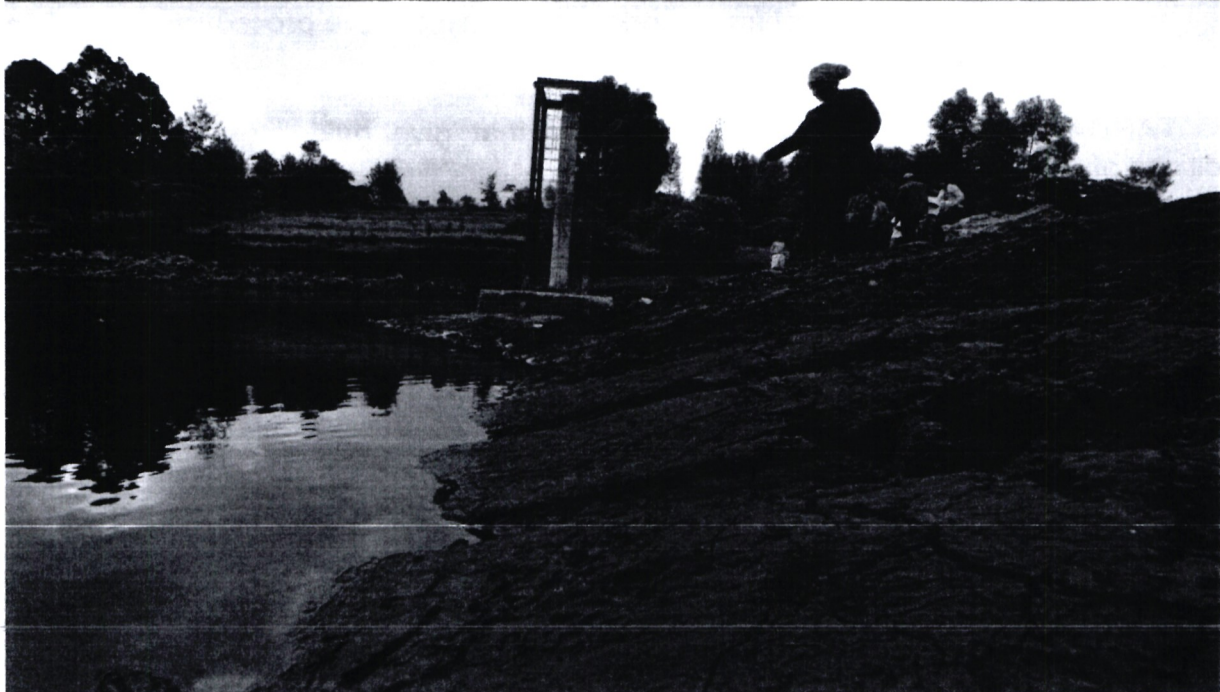
Board members visit to water harvesting dam in Othaya
